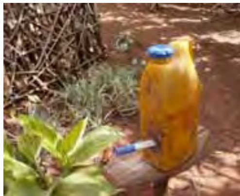
Figure 20.10 Simple handwashing facility placed conveniently outside a household latrine. (Photo: Pam Furniss)
