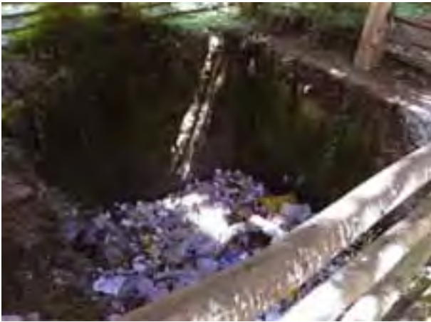
Figure 22.6 Refuse pit with a fence to prevent people or animals from accidentally falling in. (Photo: Pam Furniss)
