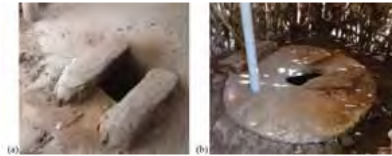
Figure 20.3 (a) Slab with raised footrest in a pit latrine. (b) Round cement slab with keyhole-shaped squat hole and footrests. Note also the vent pipe and lid. (Photos: Pam Furniss)
