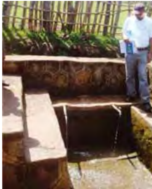
Figure 15.7 A protected spring. Note the concrete retention wall with two delivery pipes and the surrounding fence. (Photo: WaterAid in Ethiopia)
