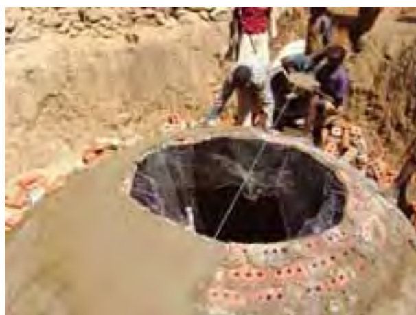
Figure 19.6 An anaerobic digester under construction. (Photo: WaterAid in Ethiopia)
