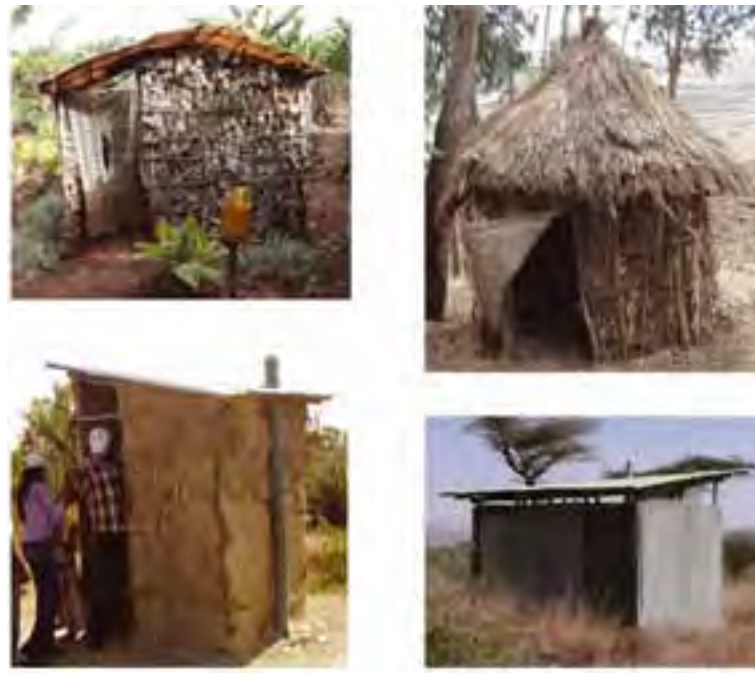
Figure 20.2 Pit latrine superstructures can be built of different materials as long as they provide privacy and protection from the weather. (Photos: Pam Furniss, Abera Kumie, Worku Tefera)
