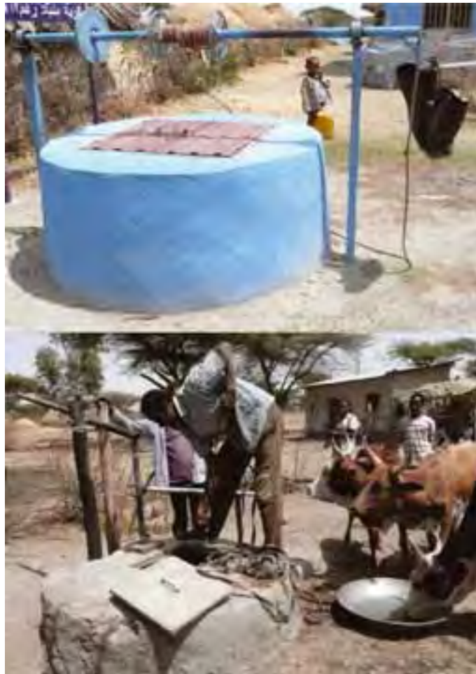
Figure 15.6 Two wells with concrete protection. Note the removable covers. (Photos: Pam Furniss)
