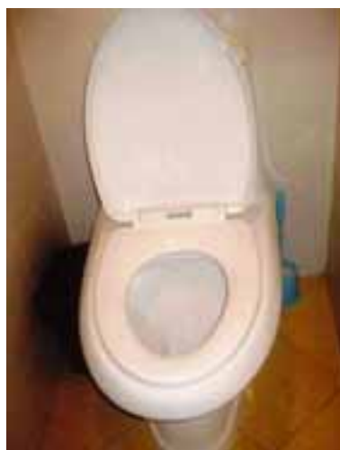
Figure 18.6 Water closet (WC) toilet. (Photo: Worku Tefera)
