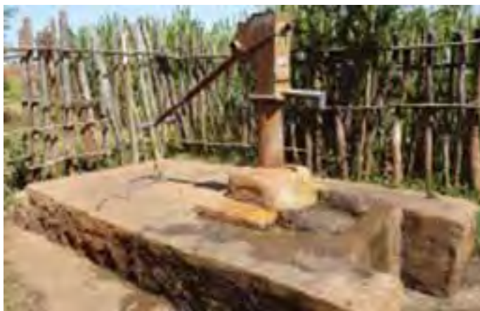
Figure 15.5 Protected handpump over a dug well. Note the concrete surround and the fence to keep out animals. (Photo: Pam Furniss)
