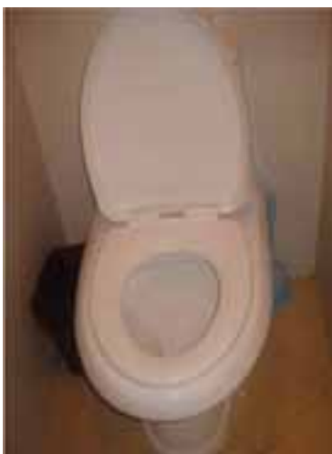
Figure 20.7 Cistern flush toilet: in this example, the cistern or tank is behind the raised lid. (Photo: Worku Tefera)
