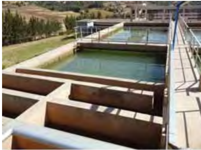
Figure 14.10 Sedimentation tank at a municipal water treatment works. (Photo: Pam Furniss)
