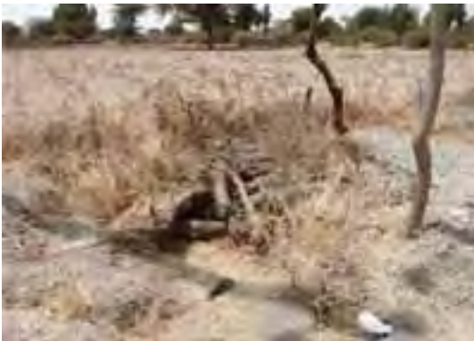
Figure 19.1 An open latrine with no privacy for the user and an insecure cover of logs – an example of unimproved sanitation. (Photo: Pam Furniss)
