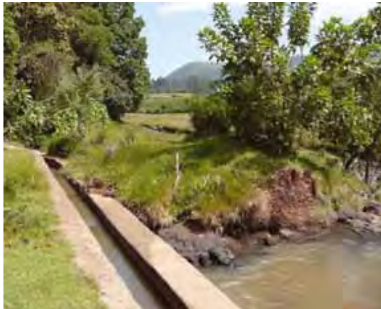
Figure 17.3 An irrigation channel carries water from the river to the fields. (Photo: Pam Furniss)
