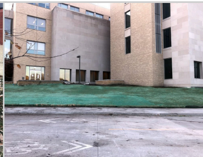
After construction of the business building addition, hydromulch was used to protect the surface and help establishment of the new grass seed. Photo credit Amber Anderson
