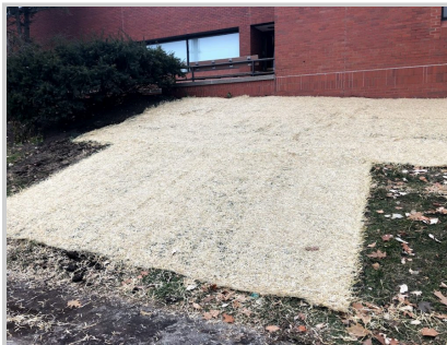
This mat is used to help protect the soil surface and keep seed in place during establishment. Photo credit Amber Anderson
