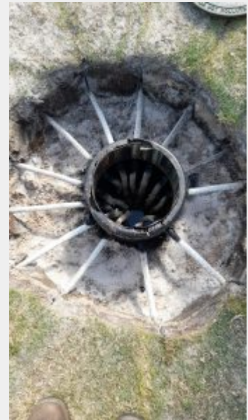
Passive Capillary drainage in a saturated soil in Florida. Picture by: Arturo Flores.
