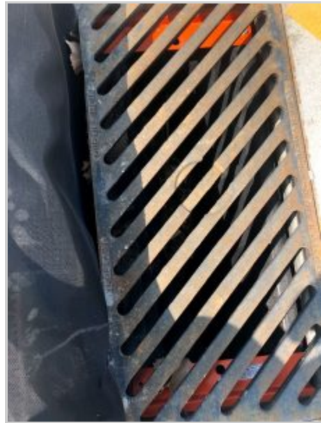
During construction, this black bag was used to capture sediment and any other materials that would have otherwise moved into the storm sewer and water system. Photo credit: Amber Anderson.
