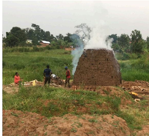
Clay being harvested near Kamuli, Uganda, is being made into bricks in this oven on site. Photo credit: Amber Anderson.
