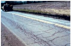
Figure 3.10 - Alligator Cracking in Asphalt Pavements
