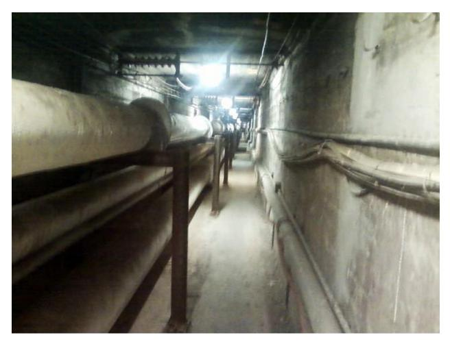
Figure 16.8 - Illustration of a Small Utilidor on a University Campus
