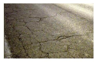
Blocks are interconnected cracks that divide the pavement into rectangular pieces. Block cracking usually indicates that the asphalt has hardened significantly.
