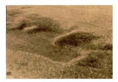
Figure 3.12 - Distortions in Asphalt Pavements
