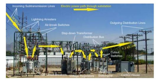
Figure 15.8 -Components of a Typical Substation
