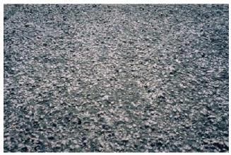
Figure 3.16 - Weathering and Raveling in Asphalt Pavements
