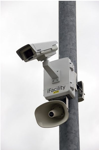
CCTV camera and iFacility IP Audio speaker on a pole by RickySpanish used under CC-BY-SA 4.0
