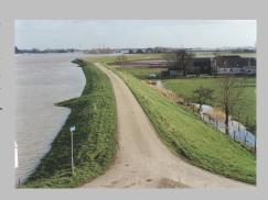
Figure 5.1: The river dike between Kesteren and Opheusden, the Netherlands, during extreme water levels of the river Nederrijn in 1995.
