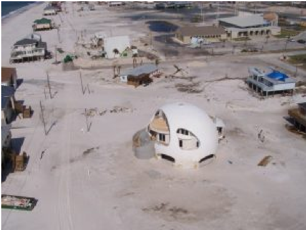
Photo 41: Dome house survived hurricane: Pensacola, Florida. Creative Commons.
