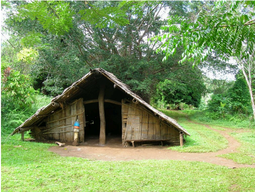
Photo 43: Traditional cyclone resistant Nakamal structure on Vanuatu. Photo by Andrew Grey. Creative Commons
