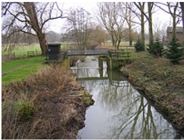
A river Gauging Station, that measures river discharge.
