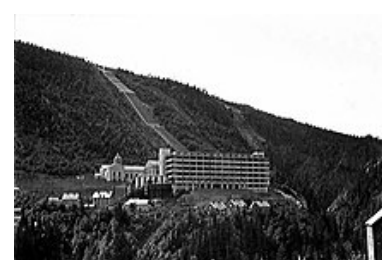
The Vemork Hydroelectric Plant in 1935, the source of heavy water.
