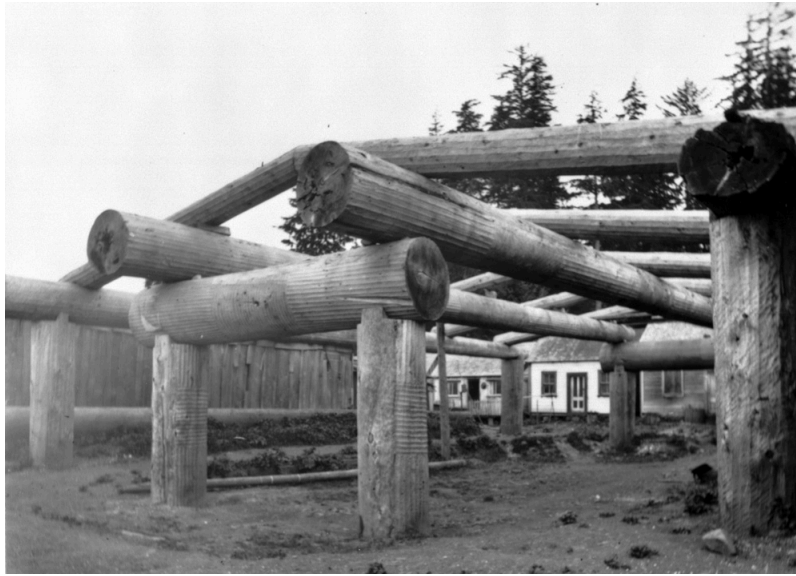
Figure 7.8 ▲ The framework of a large house with fluted beams in the Kwakiutl village of Mamalilikulla on Village Island, near Yalis (Alert Bay). Photographer Unknown. PN 1068, courtesy of the Royal BC Museum (1912).
