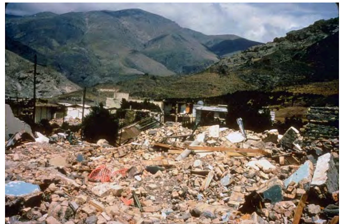
Figure 9.29: Example of devastation on unreinforced masonry by seismic motion.
