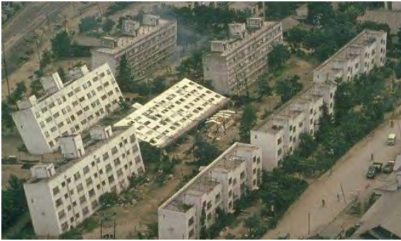
Figure 1.20: Buildings toppled from liquefaction during a 7.5 magnitude earthquake in Japan.
