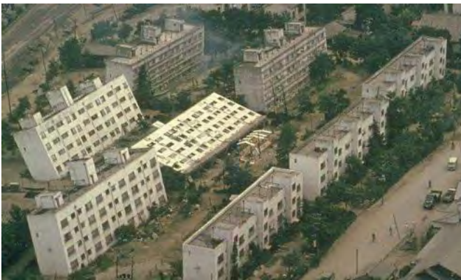
Figure 9.32: Buildings toppled from liquefaction during a 7.5 magnitude earthquake in Japan.
