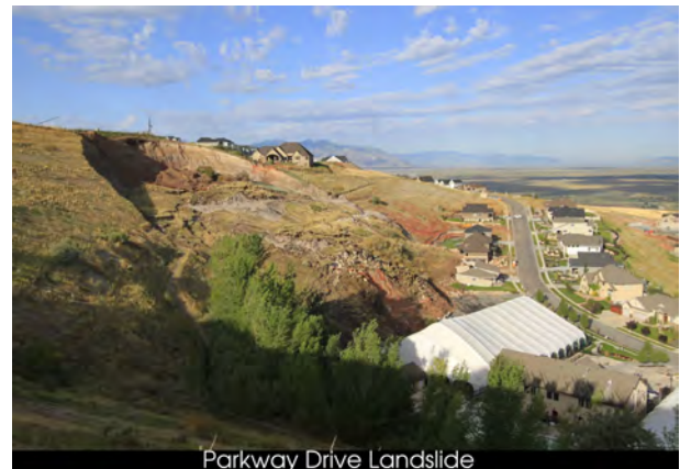
Figure 10.16: Scarp and displaced material from the North Salt Lake (Parkview) slide of 2014.
