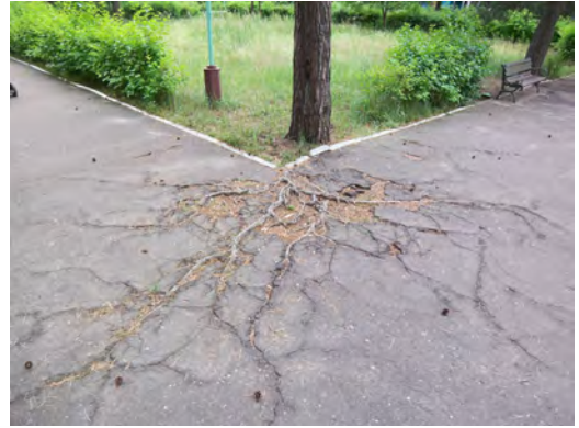
Figure 5.7: The roots of this tree are demonstrating the destructive power of root wedging. Though this picture is a man-made rock (asphalt), it works on typical rock as well.
