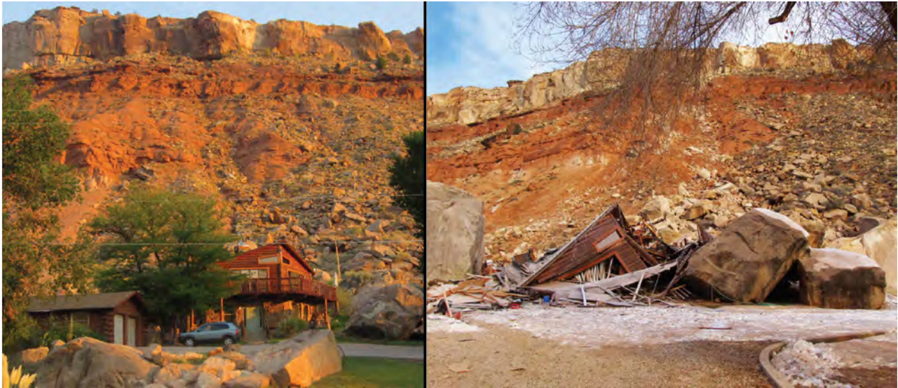
Figure 10.15: House before and after destruction from 2013 Rockville rockfall.
