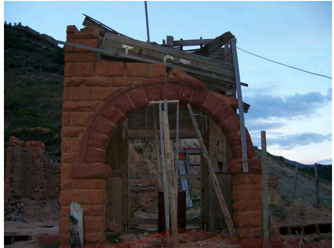
Figure 9.34: Schoolhouse in Thistle, Utah destroyed by a landslide.
