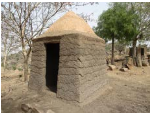
Square shaped guest hut at the Hidi's palace ongoing reconstruction.
