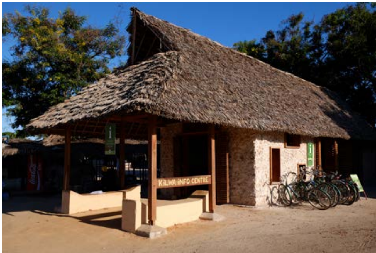
Completed Kilwa information centre © CRAterre / N. Sanchez Munoz
