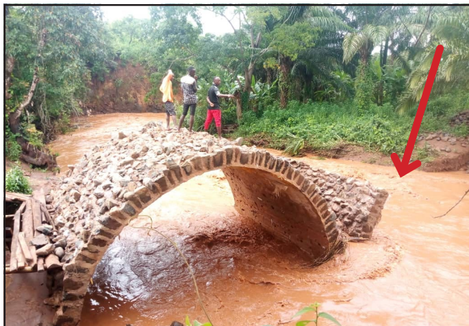
kielelezo 46 : Left: Floods carry debris from upstream. This debris gets stuck on the formwork in further increasing the pressure on the wooden structure with the risk of carrying it away. Right: If there is a risk of heavy flooding, additional anchoring of the formwork is required. Timber poles stretching across from one abutment to the other will hold the formwork together. They are the basis for additional poles which are nailed parallel with the abutments in the river bed. A large opening should be left in the middle where the debris can pass.
