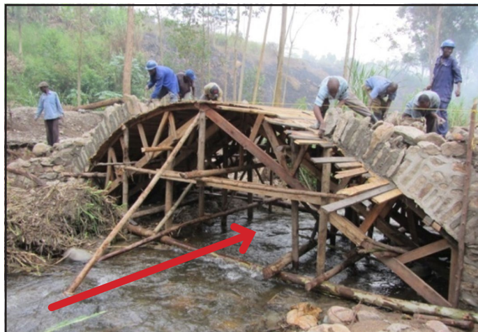
kielelezo 46 : Left: Floods carry debris from upstream. This debris gets stuck on the formwork in further increasing the pressure on the wooden structure with the risk of carrying it away. Right: If there is a risk of heavy flooding, additional anchoring of the formwork is required. Timber poles stretching across from one abutment to the other will hold the formwork together. They are the basis for additional poles which are nailed parallel with the abutments in the river bed. A large opening should be left in the middle where the debris can pass.
