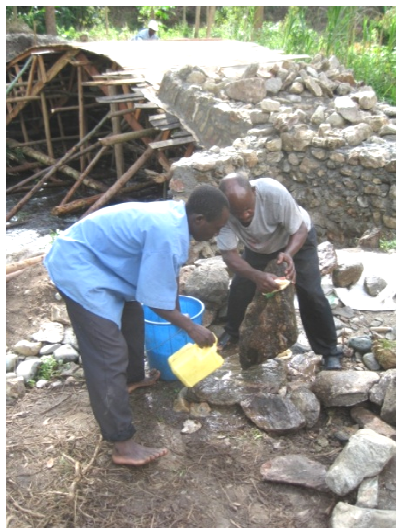
Fig. 45: The use of a gauged batch box and ruler is a precondition for producing quality mortar. Basins and wheel barrows should not be used as it is difficult to control the exact amounts.
