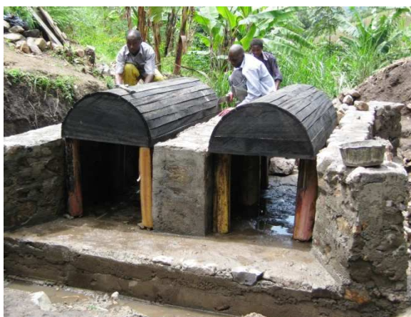
Fig. 33: The moulds for culverts are standard (here 80 cm diameter and 2 metres long). They can be re-used many times. The culvert size can be adjusted in function of the site conditions (banks, water flow) by increasing the abutment height or having multiple structures.
