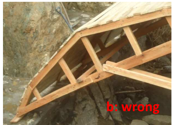
Fig. 27: The correct curve of the truss in a function of the span and the type of arch is important. Many carpenters struggle with the principle and the process will need technical guidance. A: correct shaped formwork. B: wrong formwork consisting of a set of straight lines. This latter formwork had to be demolished.
