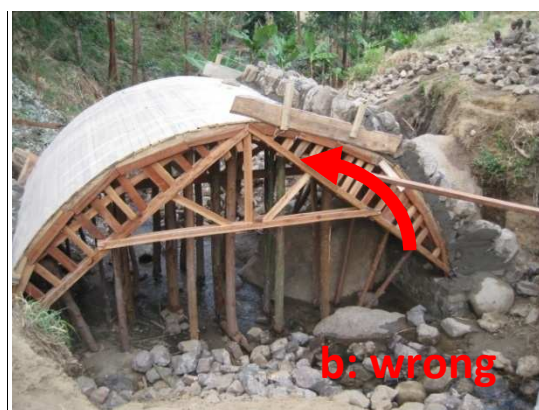
Fig. 41: For stability reasons, the bridge is built symmetrically, stepwise from both sides at the same time (a). It is dangerous to construct only one side first (b). The structure is not secure until the arch is closed in the middle.
