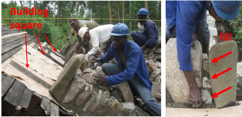
Fig 38: Left: Building squares show the right position of the stones during each phase of the arch construction. Right: It is of utmost importance to fill all gaps between the stones. Small stones will be added to the mortar to reduce cement costs and increase strength.
