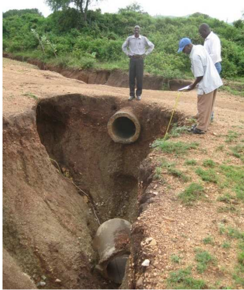
Fig 3: Eroded road due to insufficient drainage capacity of the culverts
