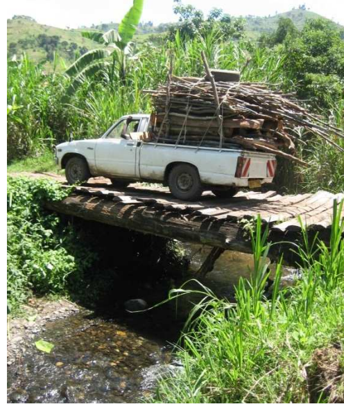
Fig 4: Timber log bridges have limited span (10 to 12m) and lifespan (4 to 10 years).
