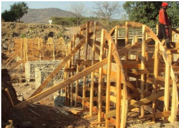
Fig 32: This formwork was constructed on site during the dry season. The span of the bridge was 50 metres and consisted of 5 arches. A rope was used to get the curved shape. The pictures are a courtesy of Rashid Mtamila/Tz.
