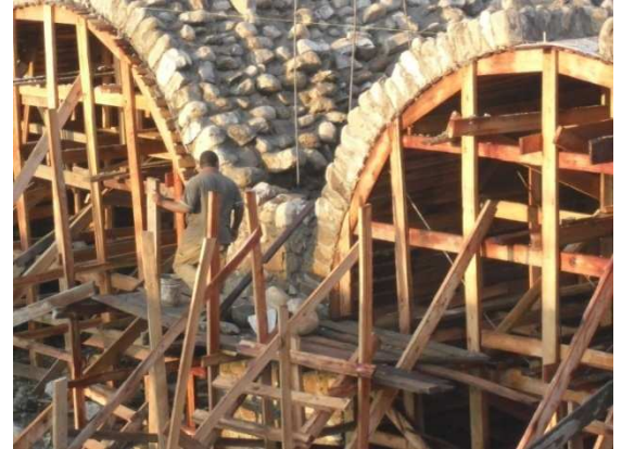
Fig 32: This formwork was constructed on site during the dry season. The span of the bridge was 50 metres and consisted of 5 arches. A rope was used to get the curved shape. The pictures are a courtesy of Rashid Mtamila/Tz.
