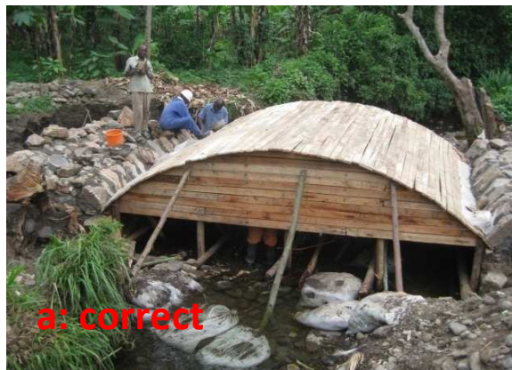
Fig. 27: The correct curve of the truss in a function of the span and the type of arch is important. Many carpenters struggle with the principle and the process will need technical guidance. A: correct shaped formwork. B: wrong formwork consisting of a set of straight lines. This latter formwork had to be demolished.
