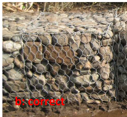
Fig 43: If not properly installed, gabions often collapse fast (a). This example started sagging after the first flood and had to be redone. Before the gabions are placed at the river banks, large stones will be rammed in as support basis to avoid early scoring under the gabion. The stones are carefully placed in the cage to avoid damaging the galvanized coating. The craftsmen will look for a good bond between the stones (b). The stone volume in the cage is 100% self supporting. There is no pressure of the stones on the cage. All cavities are filled with small stones and river sand. The gabions are filled in such way, that if walking on them, the stones should not move (c). Half way the filling, wires are tied to across the cage to reinforce the gabion
