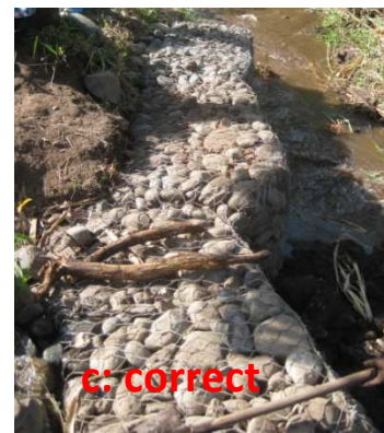
Fig 43: If not properly installed, gabions often collapse fast (a). This example started sagging after the first flood and had to be redone. Before the gabions are placed at the river banks, large stones will be rammed in as support basis to avoid early scoring under the gabion. The stones are carefully placed in the cage to avoid damaging the galvanized coating. The craftsmen will look for a good bond between the stones (b). The stone volume in the cage is 100% self supporting. There is no pressure of the stones on the cage. All cavities are filled with small stones and river sand. The gabions are filled in such way, that if walking on them, the stones should not move (c). Half way the filling, wires are tied to across the cage to reinforce the gabion
