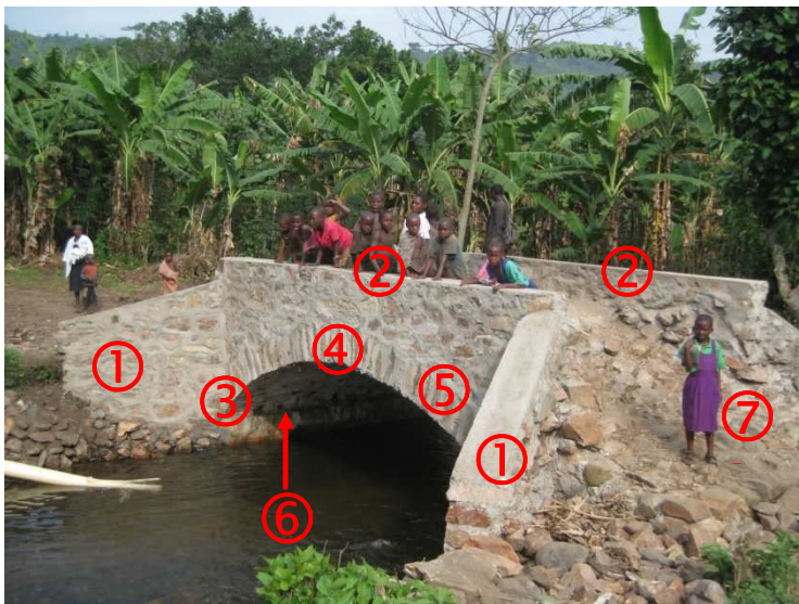
Fig 10. Vocabulary of arch bridges
