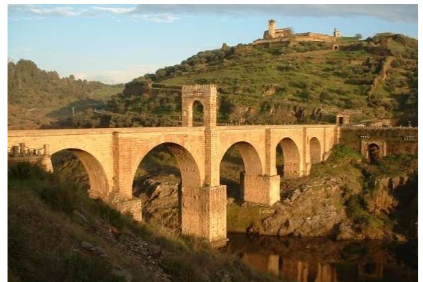
Fig 5: Roman stone arch bridge built over the Tagus River at Alcántara, Spain between 104 and 106.AD (Total length: 194m, longest span: 28m) Picture: courtesy Wikipedia.
