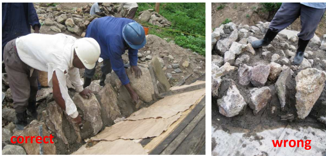
Fig 39. The quality of the craftsmanship is of extreme importance for the strength of the arch. Left: Good bond and proper positioning of stones. Right: poor stone masonry that will result in a weak structure.
