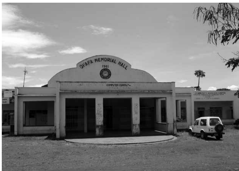
Figure 3.2. Ofafa Memorial Hall, Kisumu. Photo by author.
