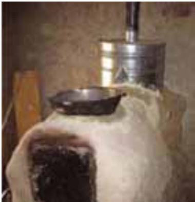
Figure 4.5 A flue attached to an oven prevents smoke and fumes from polluting the air in a rural house.
