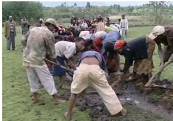
Figure 9.1 Community members digging a ditch to drain mosquito breeding pools. (Photo: Dr Daddi Jima)
