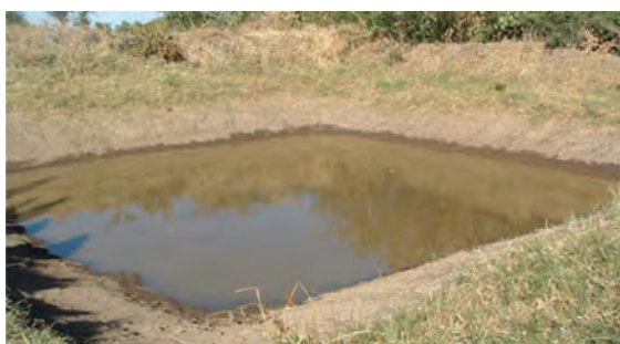
Figure 9.8 Steepening shorelines can help to prevent mosquitoes from breeding. (Photo: Dr Yemane Ye-ebiyo Yihdego)
