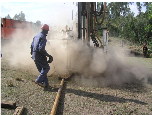
(f) Down-the-hole hammer
