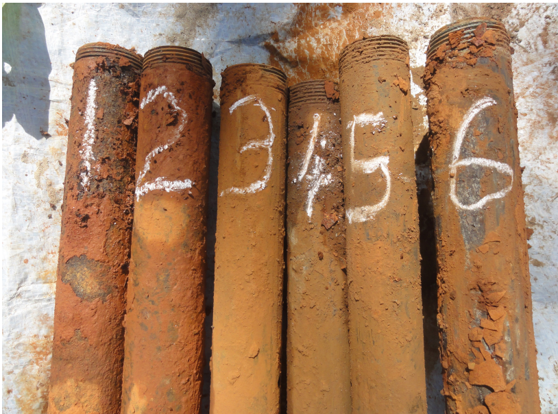
Figure 5.7 Corrosion of India Mark II galvanized rising main in northern Uganda
