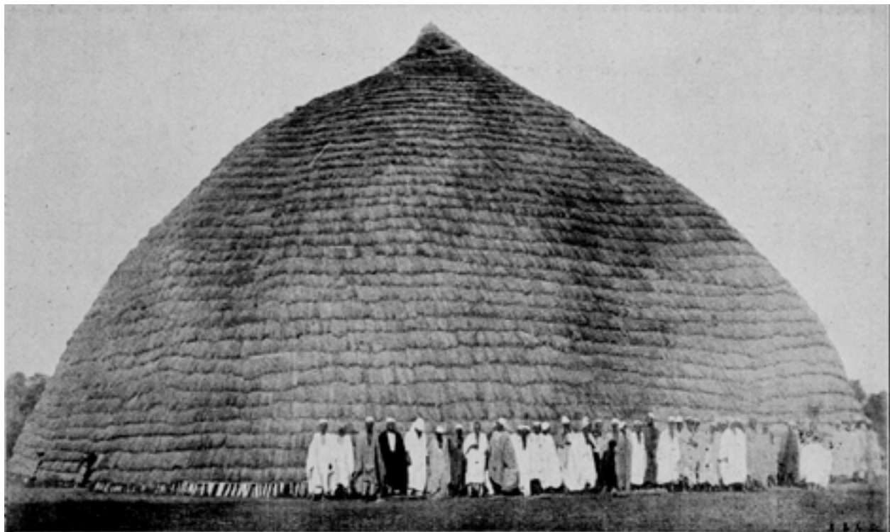
FIG. 652. The Dinguiraye mosque was the largest of the 18th and 19th-century Fulani mosques in Guinea. Its square earthen interior was completely masked by the great roof, which was 164' in circumference. Fulani male builders, Dinguiraye, Guinea, 19th century. Photo from Lucien Marie Francois Famechon's book, Notice sur la Guinée française (Paris: L'Exposition, 1900). Public domain.
