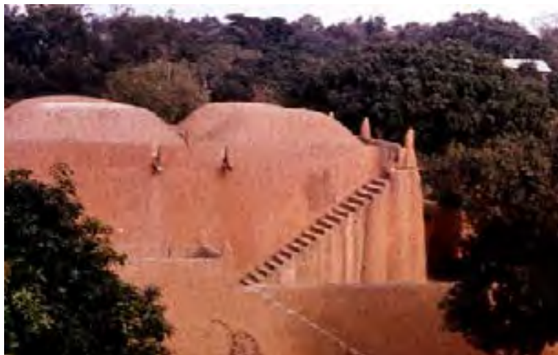
FIG. 670. This full-scale reproduction of the early 19th-century Zaria Friday Mosque built by Mallam Mikaila stands in the Museum of Traditional Nigerian Architecture, Jos. The stairs lead up to the roofline for the muezzin to chant the public call to prayer; the roof's six low "domes" are visible. Photo by Kathy Curnow, 1987.
