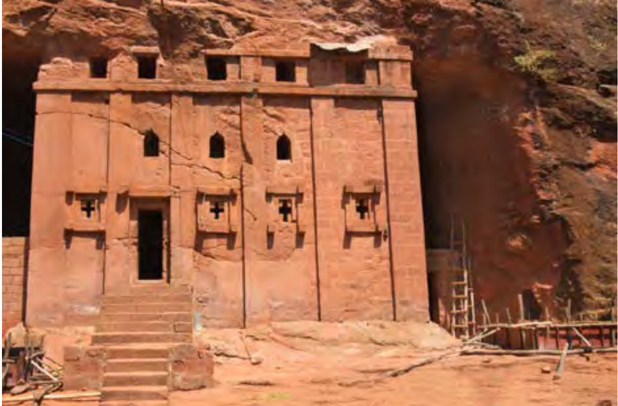
FIG. 606. The Biete Abba Libanos church has dressed blocks on its right side; these seem to be an early repair or structural choice. Male builders, Lalibela, Ethiopia, 12th-13th century. Photo by A. Davey, 2007. Creative Commons CC-BY 2.0.
