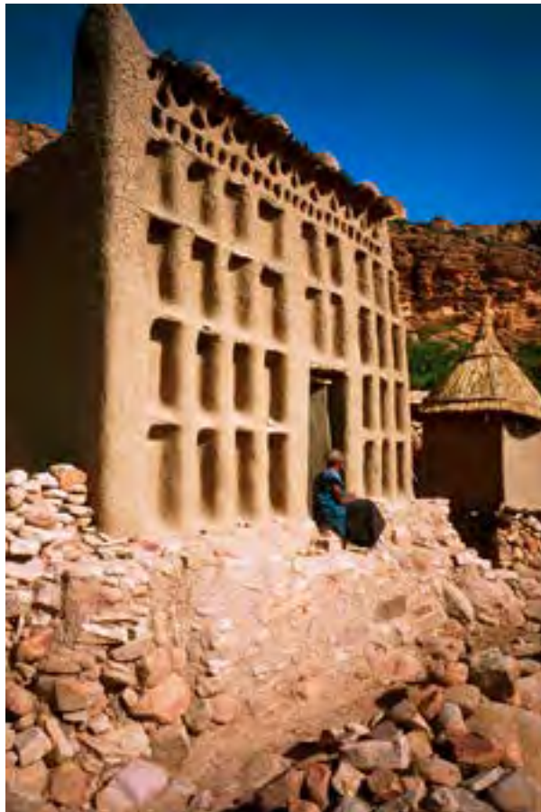
FIG. 428. This ginna , or lineage head's house, is marked by distinctive niches on its facade. Not all ginna , however, have this architectural trait. Photo by John Spooner, 2002. Creative Commons CC BY 2.0.
