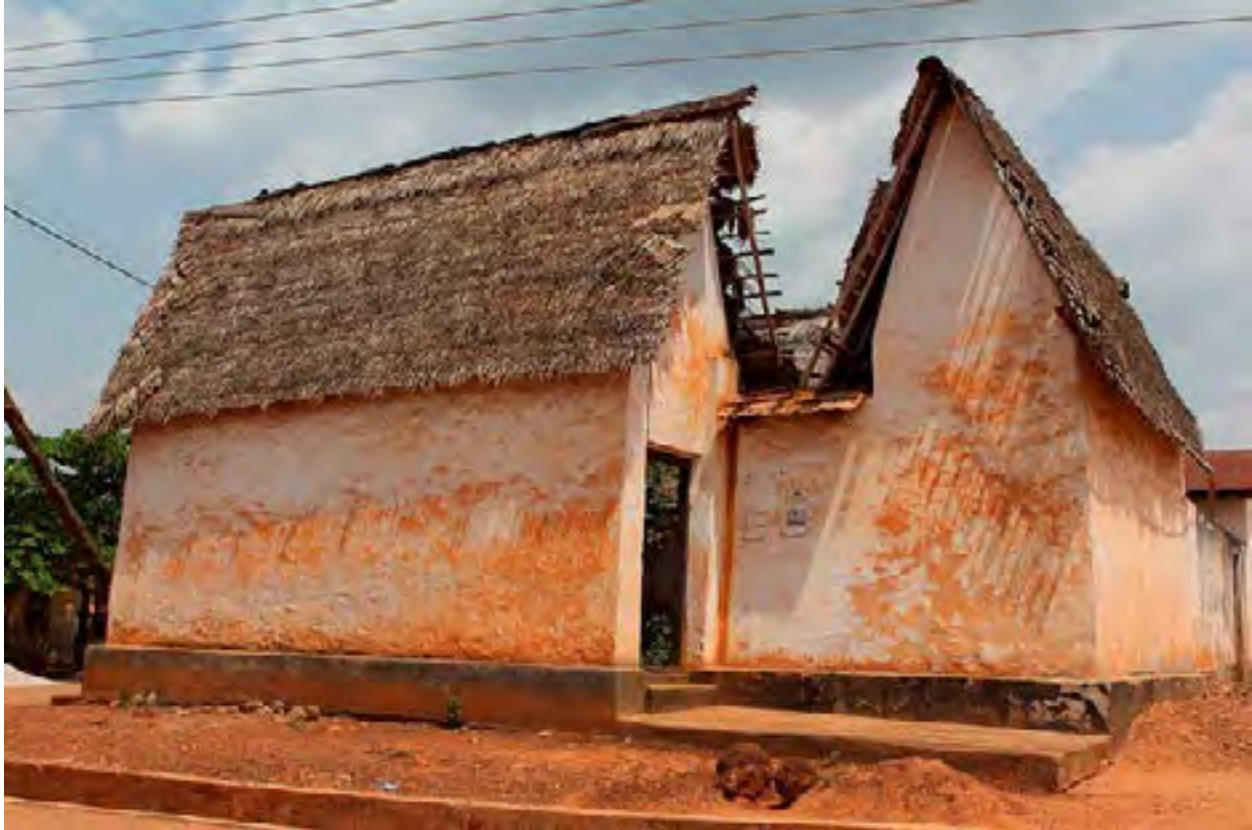
FIG. 824 This shrine follows the form of traditional Asante domestic architecture, the high-pitched thatched roofs designed to shed rain. Photo of Besease shrine by Carsten ten Brink, Ghana, 2012. Creative Commons BY-NC-ND.
