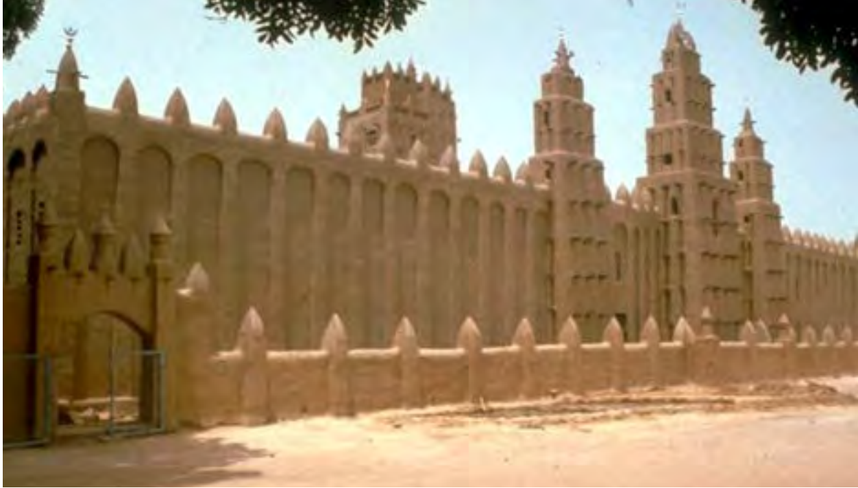
FIG. 686. In 1973, architect/mason Lassine Minta completed the expansion and reconstruction of the Niono Main Mosque in Mali's Segou region with a team of masons from Jenne. It won the Aga Khan award for architecture a decade later. It mimics the Jenne main mosque in numerous respects, but its stepped minarets depart in form from Jenne's towers, and it displays greater regularity and symmetry. Image courtesy of Nasser Rabbat of the Aga Khan Program at MIT, 2002. Creative Commons CC BY-NC-SA 2.0. Right: The minaret of a northern Algerian mosque formerly in El-Attaf, also topped by an ostrich egg. Image from H. B. Tristram, The Great Sahara: Wanderings south of the Atlas Mountains . London: Murray, 1860, opp. p. 170. Public domain.
