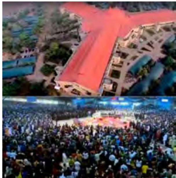
FIG. 590. The Faith Tabernacle, headquarters of the Pentecostal Living Faith Church Worldwide International, holds 50,000 people in a structure with industrial leanings, somewhat like a trade show exposition center. It covers approximately 70 acres, set within a much larger complex. An expanded structure that will hold twice as many is planned. Lagos, Nigeria, 1998-1999. Single frames from Moses Ntam's 2016 video, "Living Faith Church, Faith Tabernacle: A City Without Walls."
