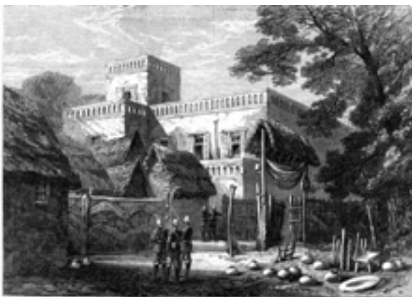
FIG. 826 The Asantehene's stone structure, completed in 1822, stood in the midst of traditional buildings within the vast palace complex. Like traditional Akan structures, it was built around a courtyard, but its other architectural features are solely European in impulse. Fante male builders, Ghana, 1822. Image from Illustrated London News , Apr. 25, 1874.
