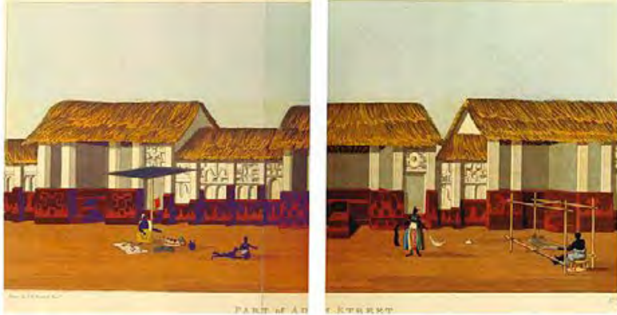
FIG. 825 View of Adum Street, near the palace. Relief decorations decorate the surfaces of the buildings; the base is left the natural red of the clay, so splashing in the rainy season won't change its color, while the rest of the house is painted with "chalk"—white kaolin clay. Watercolor from Thomas Edward Bowdich's Mission from Cape Coast Castle to Ashantee (London: John Murray, 1819), plate 9. Public domain.
