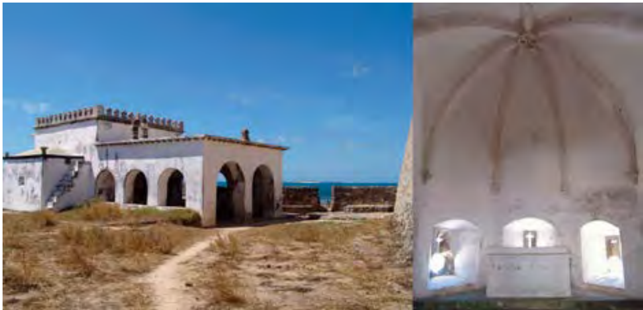
FIG. 578. The chapel of Our Lady of Baluarte, built by the Portuguese on Mozambique Island in 1522, is the oldest standing Christian church south of the equator. Its simplified stone structure—much less elaborate than contemporaneous churches in Portugal—includes a vaulted interior, arched porch, and a rain catchment roofing system. Photos by Spielkind at English Wikipedia, 2006. Public domain.
