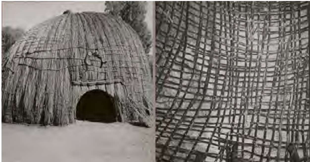
FIG. 716 Exterior and inner roof of a Zulu indlu. Photo by Jean-Erick Pasquier, Orange Free State, South Africa, 1969. © Musée du Quai Branly, PP0075781.2.
