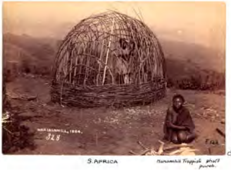
FIG. 715 A Zulu man preparing the armature for a house, 1894. Pitt Rivers Museum, University of Oxford, 1998.160.13.4. Creative Commons CC BY-NC-ND 4.0.
