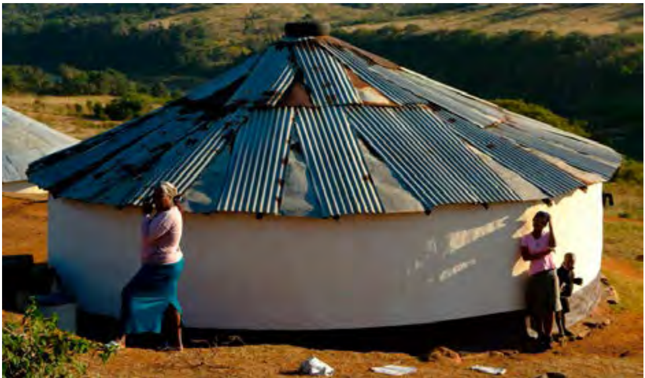
FIG. 719 Zulu whitewashed house with corrugated metal roof. Photo by Steve McNicholas, 2006. Creative Commons CC BY-NC-ND 2.0.
