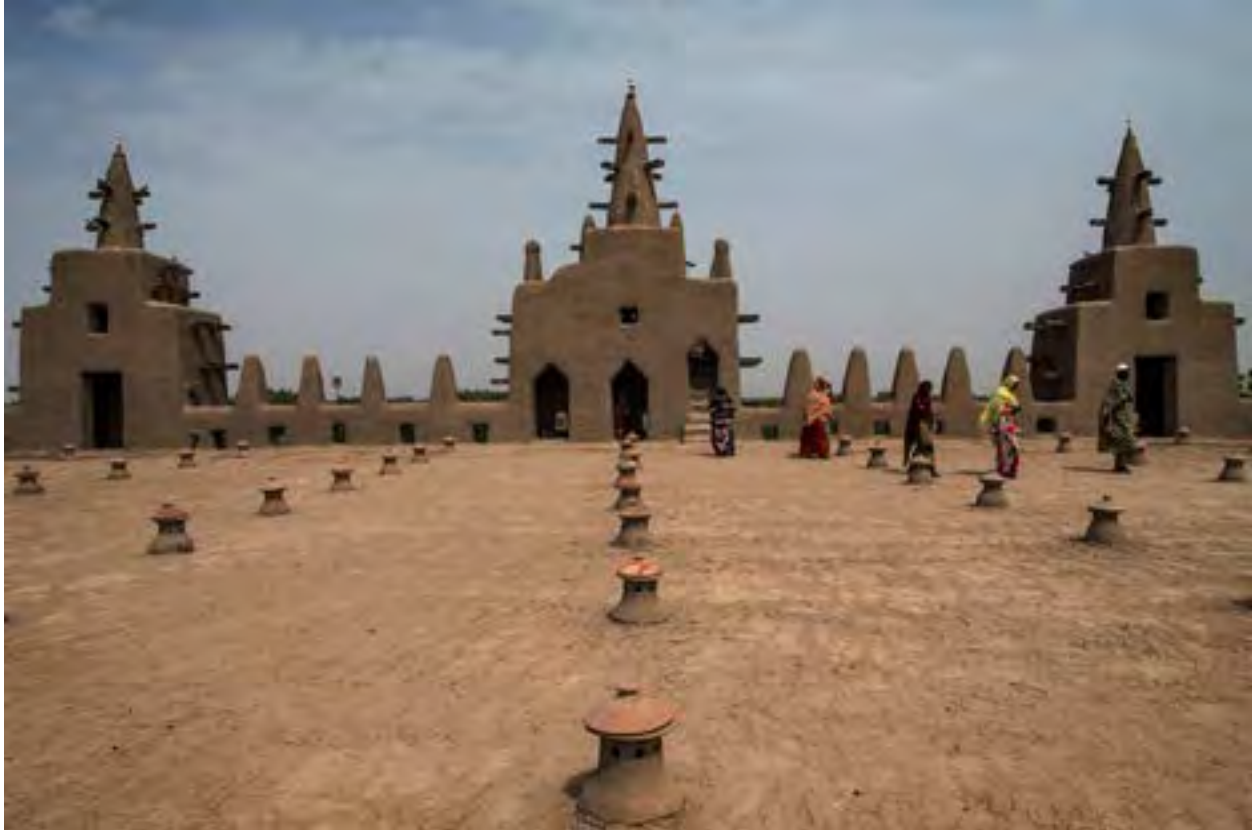
FIG. 683. The flat roof of Jenne's Main Mosque allows venting of hot air when the pot lids are removed. Photo by Marco Dormino, United Nations, 2015. Creative Commons CC BY-NC-ND 2.0.
