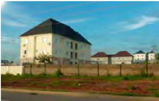
FIG. 82. Panel roofing, Abuja, Nigeria, 2012. Photo Bryn Pinzgauer. Creative Commons CC BY 2.0, cropped.
