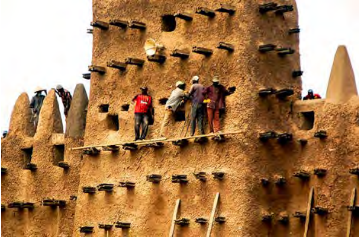
FIG. 684. The annual resurfacing of the mosque began in this section with the sarafar. Photo by Ralf Steinberger, 2009. Creative Commons CC-BY 2.0.
