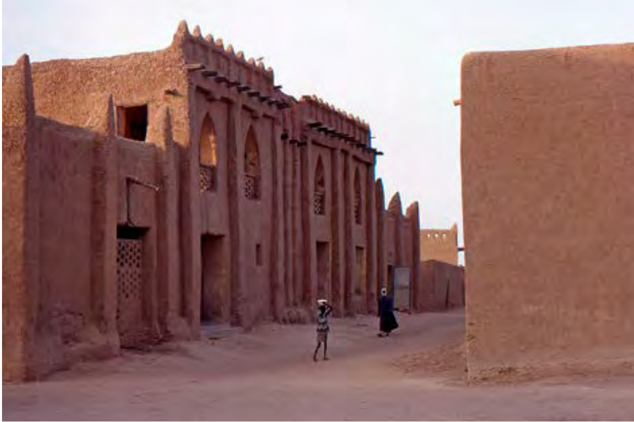
FIG. 32. A street in the town of Jenne in Mali, where masons construct the buildings, 1972. Photo by Gilles Mairet. Creative Commons CC BY-SA 3.0.
