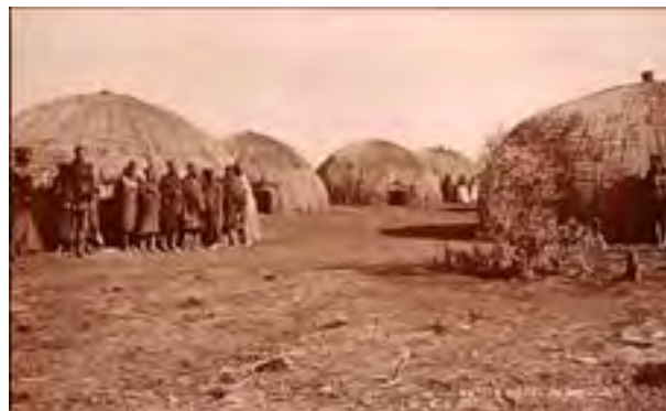
FIG. 30. Zulu families used to live in fiber houses spaced in a circular arrangement, their cattle kept in the middle. Women built the structures, binding fibers and grass over a reed support. South Africa, early 20th century. Public domain.
