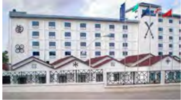
FIG. 863 The Golden Tulip Hotel in Kumase, Ghana, remodeled in 2008. Photo by ZSM, 2008. Creative Commons BY-SA-3.0.
