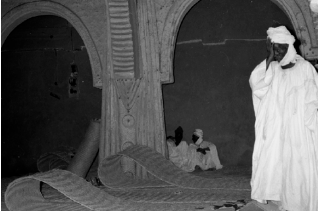
FIG. 673. Interior of the Zaria Friday Mosque, with relief ornamentation and a double arch. Mallam Mikaila, Hausa male architect, Zaria, Nigeria, 1830s-40s. Photo by Hamo Sassoon, 1930s-1970s. Pitt Rivers Museum, 2005.113.942. Creative Commons CC BY-NC-ND 4.0.
